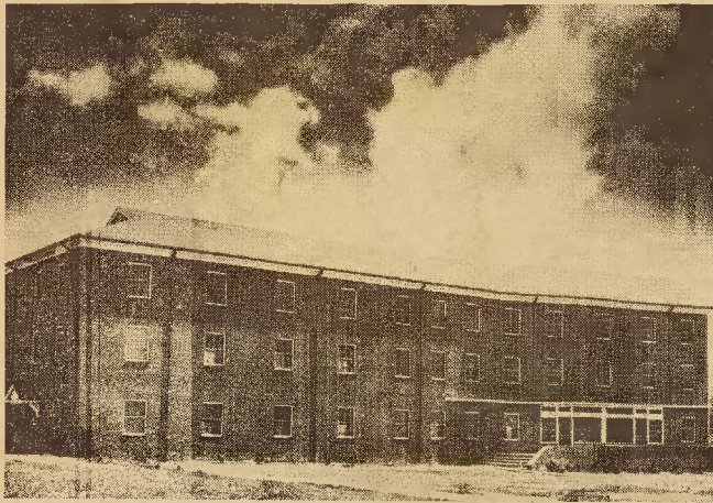
The new dormitory for women constructed by the J. A. Jones company on the campus at Brevard college will be on display at open house Sunday afternoon from 4 to 6 o'clock.
