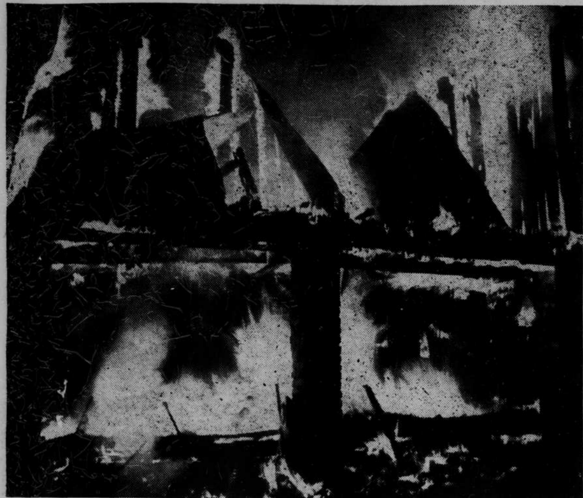
ANOTHER TRANSYLVANIA HOME was completely destroyed by fire, when the house of Mrs. Bernice Collins burned to the ground on the Tinsley road about 10:30 o'clock last Friday night. The above photo was made just as the firemen arrived on the scene and it can be quickly noted that it was impossible for
