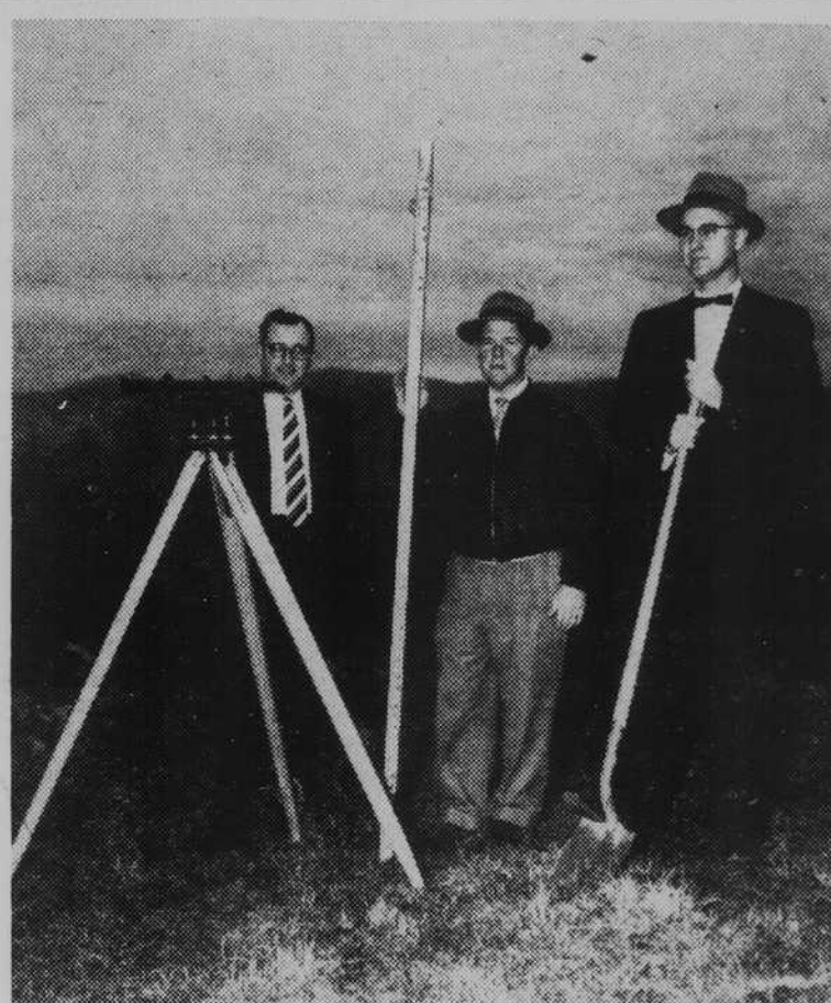
PRESIDENT ROBERT H. STAMEY , right, turns the first shovel of dirt early Tuesday morning for the new men's dormitory at Brevard college. In the center is Jack Jameson, superintendent of the construction for the J. A. Jones Construction Co., and at the left is Guy Burchfiel, dean of men and assistant to the president at the college. The new dorm will be located adjacent to Taylor hall and will house 100 men. (Times Staff Photo)
