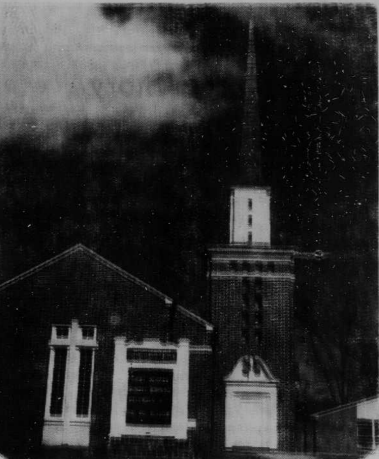
THE NEW PRESBYTERIAN church in Brevard will be used by the congregation for the first time this Sunday morning. Shown above is a picture of a portion of the new building showing the sanctuary, the steeple and part of the Sunday school rooms. The structure was built since April of this year by the Jerry Liner Construction company at a cost of approximately $160,000. With the opening of this new building, the Presbyterians begin a week of Consecration and Thanksgiving services. (Times Staff Photo)
