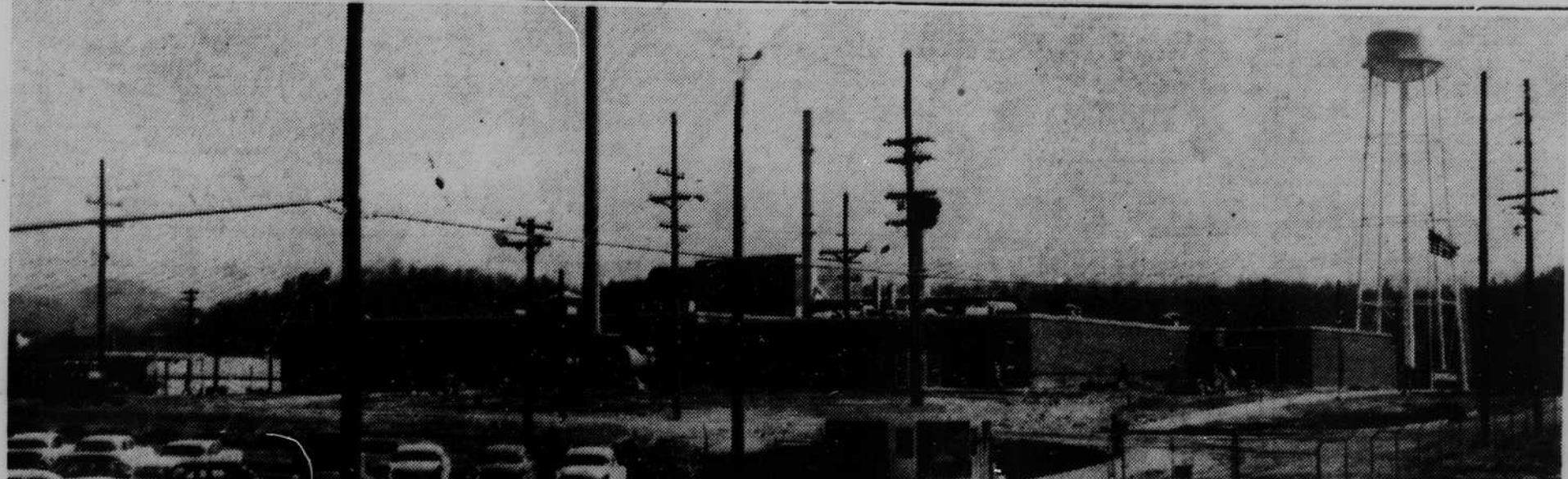
AN OVERALL VIEW of the new Du Pont silicon plant in Buck Forest is shown above. Company officials announced last week that construction of the multi-million dollar plant is "about 90 per cent" and operations are expected to start within a few months. Production
