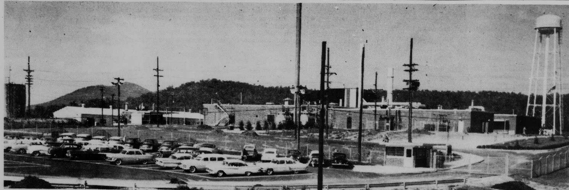
AN OVERALL VIEW of the new Du Pont silicon plant in Buck Forest is shown above. Construction has been completed, the grounds have been landscaped and the parking area and roads have been
