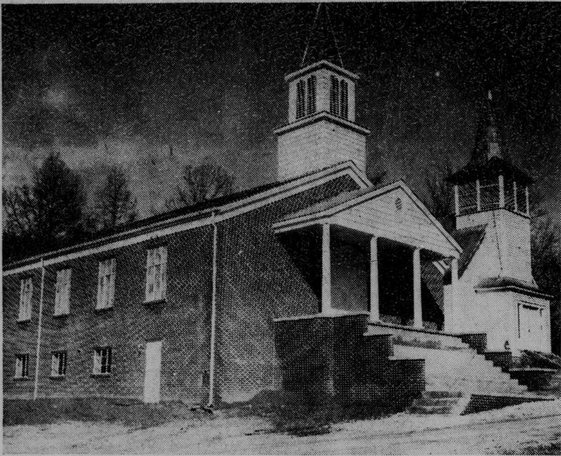
THE NEW GLADY BRANCH Baptist church, with the old church in the background, is pictured above, high atop Rocky Hill on US Highway 64. Valued at $65,000, the church is a fine example of community spirit and cooperation, Rev. Millard Brock, the pastor, states. (Times Staff Photo)
