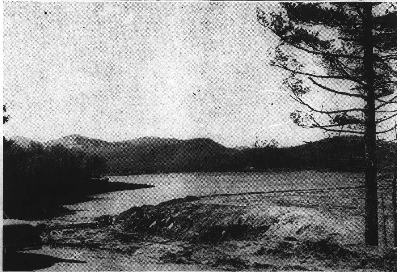
RECENT HEAVY RAINS are fast filling beautiful Lake Toxaway and this picture was made Monday from the road just above the dam. It can be noted at the left that work on the spillway around the
