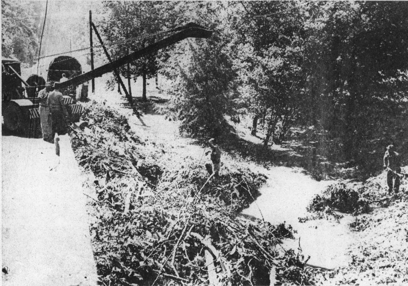
A FLASH FLOOD, caused by some five inches of rain in about an hour, did extensive damage in the Middle Fork section of upper Transylvania county last Wednesday afternoon. Highway crews are pictured above cleaning out debris below bridges along the highway. See story on page seven, second section, in this week's newspaper. (Times Staff Photo)
