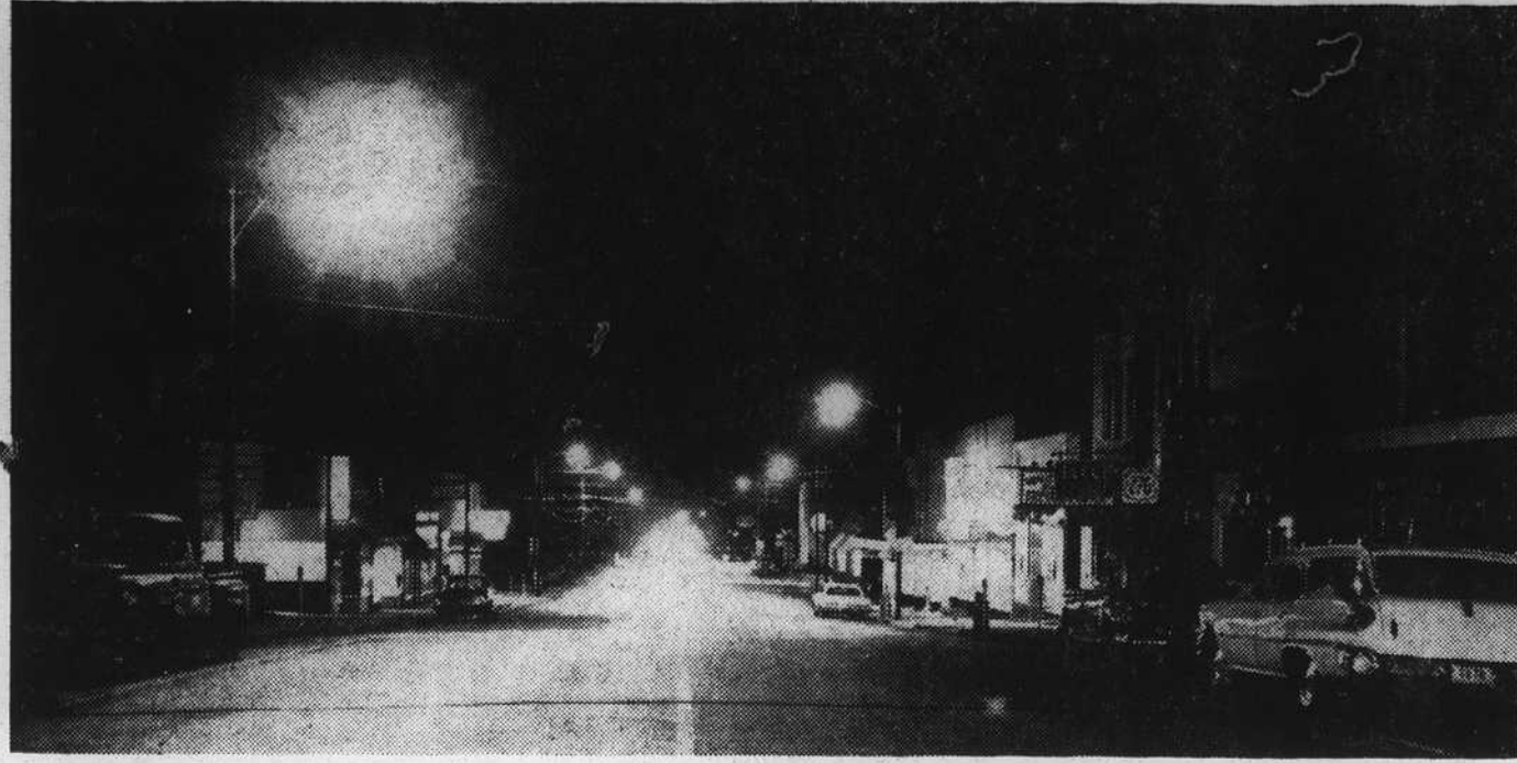
THE BRIGHTNESS of the new "White Way" in the business district of Brevard can be vividly seen in the photographs above. Last week when the work was half completed, the pictures were made. At left is the new "White Way" looking east down Main street from the square. The other picture
