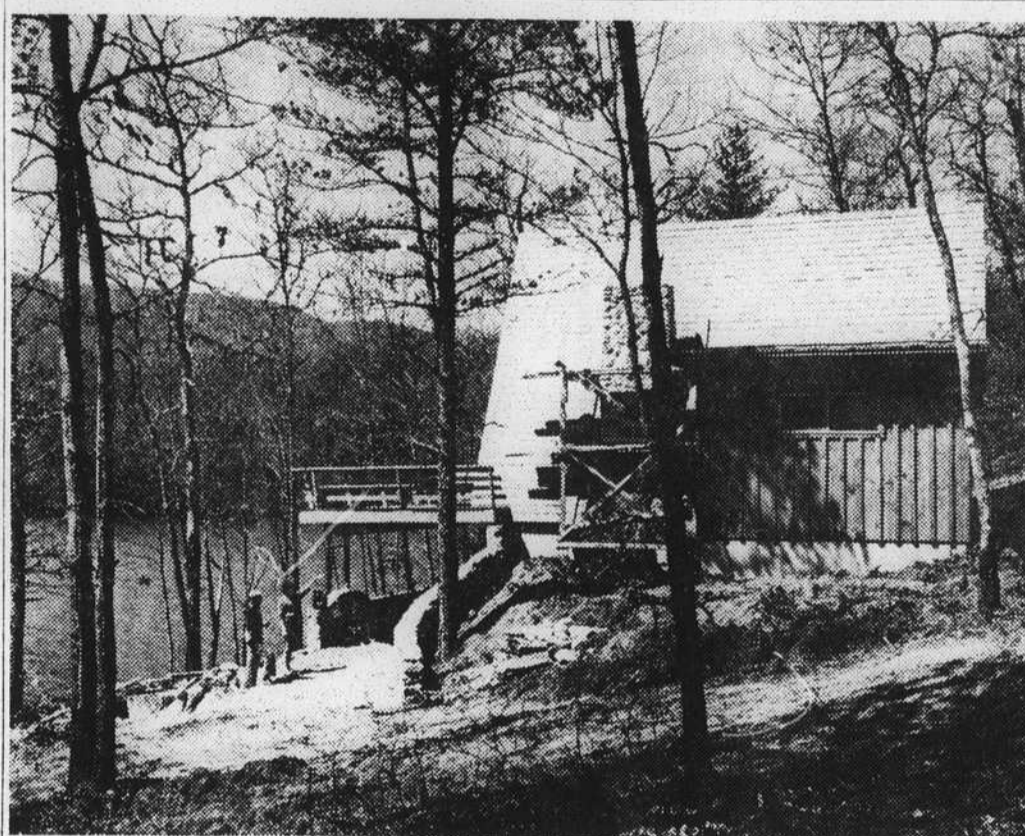
THIS LAKESIDE HOME is one of a number under construction on the shores of Lake Toxaway, in upper Transylvania. The lake, restored last year after an interval of nearly a half-century, is also the site of a new motor inn and golf course, both under construction.
