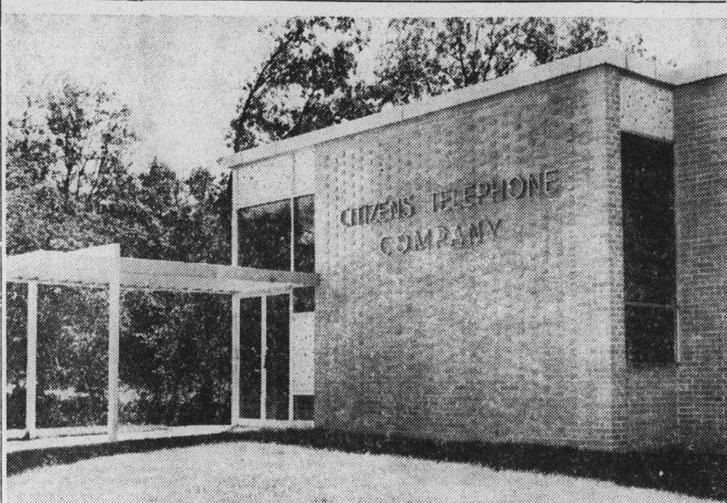
THE NEW CITIZENS TELEPHONE COMPANY is pictured above. Moving of all offices from Probert street will be completed this weekend, and the new building will be opened at 9:00 o'clock next Mon-
