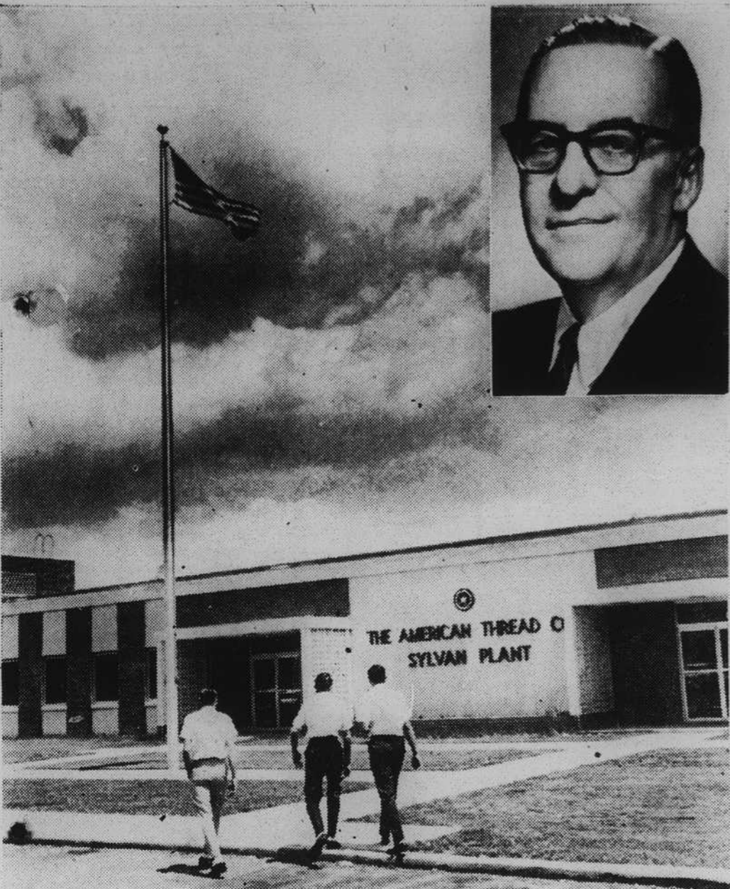
THE MODERN SYLVAN PLANT of the American Thread company at Calvert will be dedicated on Saturday, and a Housewarming from 10:00 in the morning until 4:00 in
