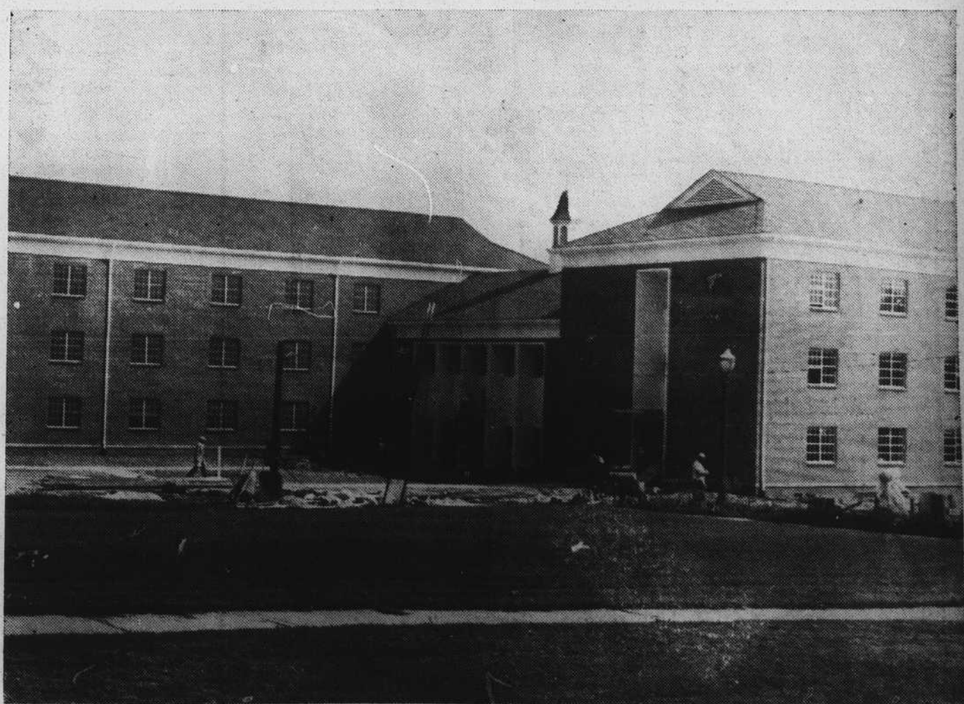
Lena Sue Beam Hall Being Completed At The College
