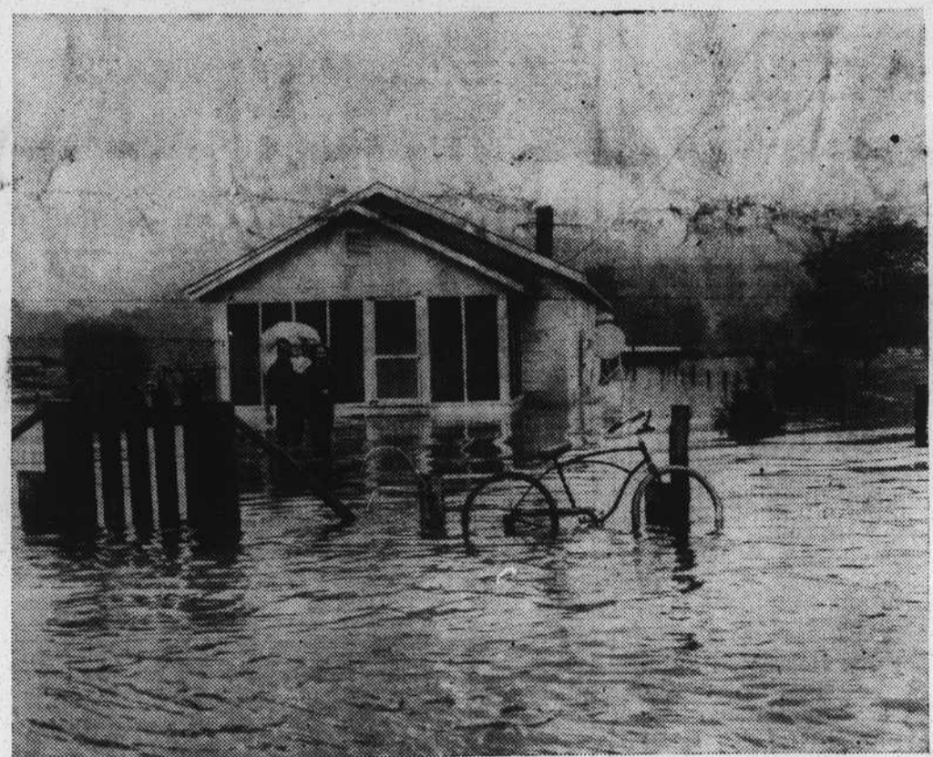
SEVERAL FAMILIES at Pisgah Forest and at Rosman were evacuated from their homes last Saturday night and Sunday morning because of the flood. Shown above is the
