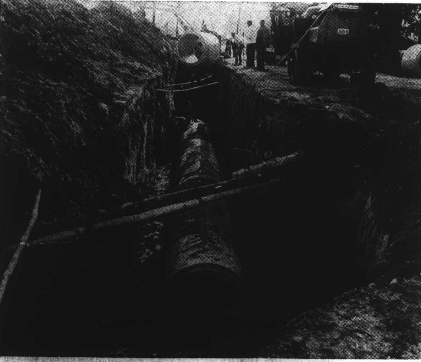
PROGRESS IS OFTEN INCONVENIENT as we are now experiencing on North Caldwell street. Shown above is a section of the new 4 foot diameter storm drain being installed to carry storm waters from along North Caldwell street and areas west of this street to Kings Creek. This section will lie about 14 feet under Caldwell street. The work is being performed by Perry Alexander Construction company of Asheville under the supervision of the State Highway Department. When complete, the project will prevent future flooding of the College Shopping Center area. The project is being jointly financed by the Town, Brevard College and the State Highway Department. (Times Staff Photo)
