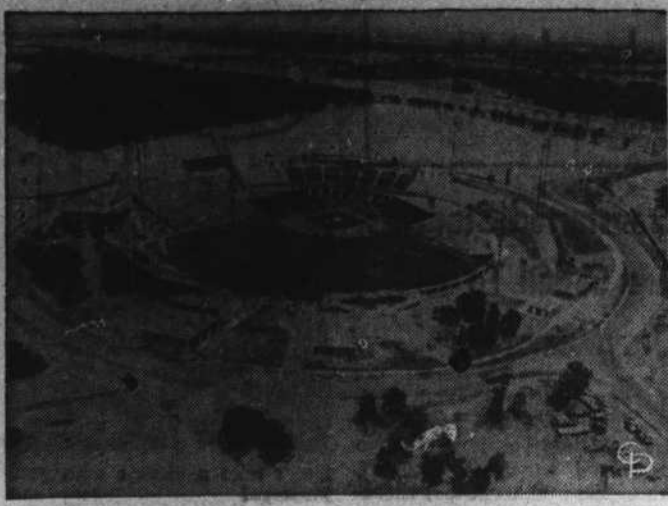
CAPITAL INVESTMENT —This is Turnpike stadium in Arlington, Tex., halfway between Dallas and Fort Worth, which will be the new home of the Washington Senators when that club is moved. The stadium now seats 22,000 and will be enlarged to seat 45,000 by April of 1973.
