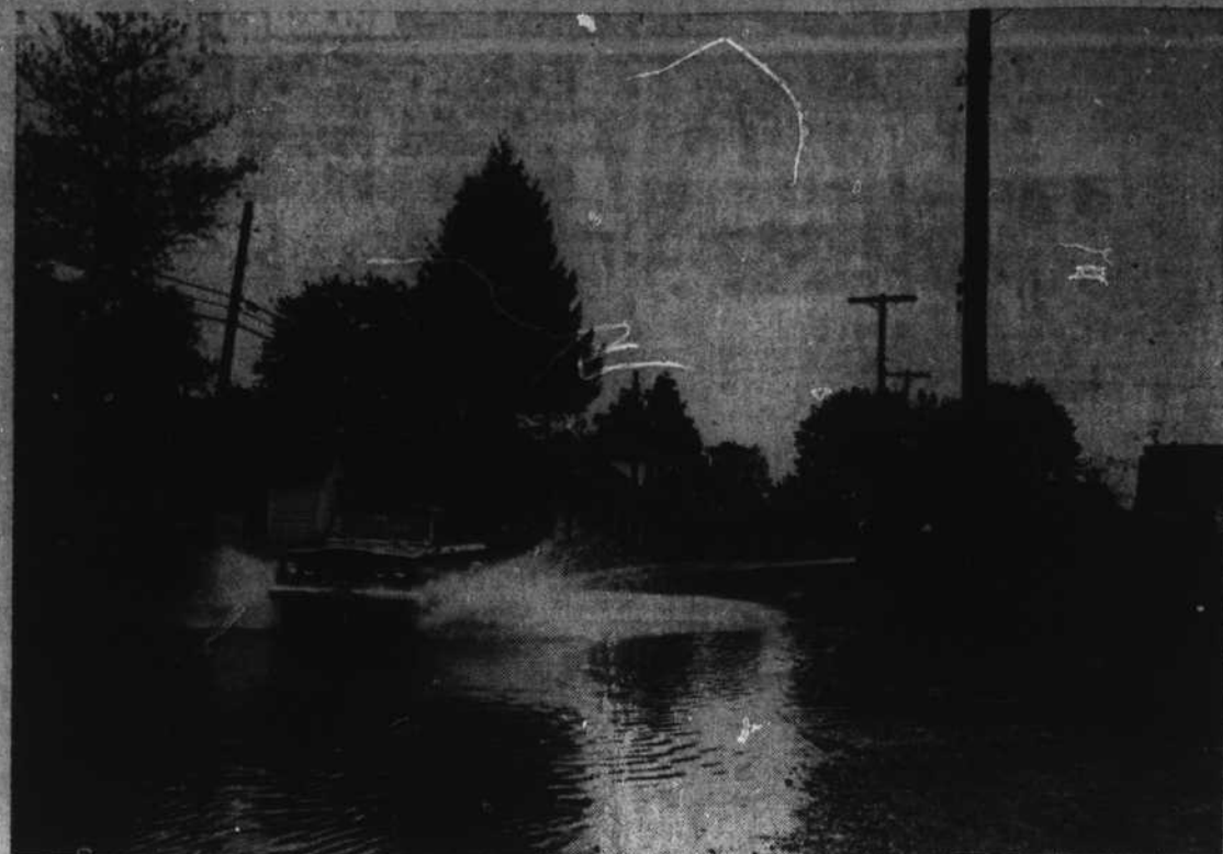
DRAINAGE PROBLEM IN PISGAH FOREST — The picture above shows the road through Pisgah Forest during the period of moderate rains in September. A storm drain, blocked by a property owner where it crosses his property, causes the water to back up across
