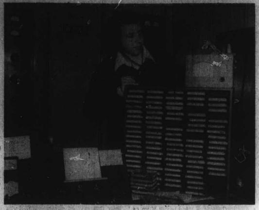
TEMPERATURE AND WIND SPEED OUTSIDE - Mike Cook, part-time announcer and engineering student at Clemson University, is shown at the read out dials of the remote - reading thermometer and anemometer he built and installed
