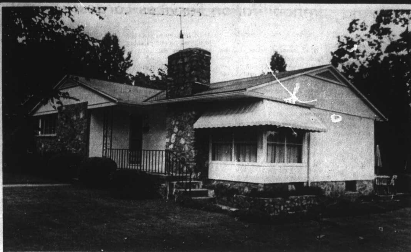
BEAUTIFULLY LANDSCAPED three-bedroom, one and one-half bath home in a convenient location. Rock fireplace in living room and Franklin fireplace in family room. Exterior recently painted. Full basement. Home in excellent condition. $37,500.
