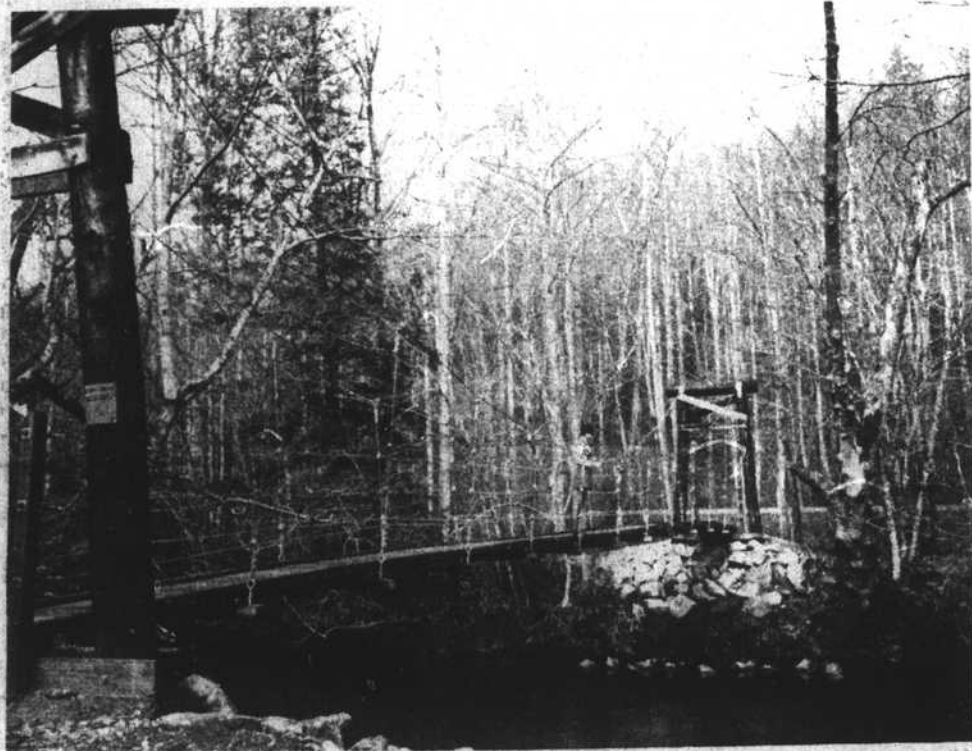
New swinging bridge, just completed on Davidson River will provide entrance to the Art Loeb Trail.
