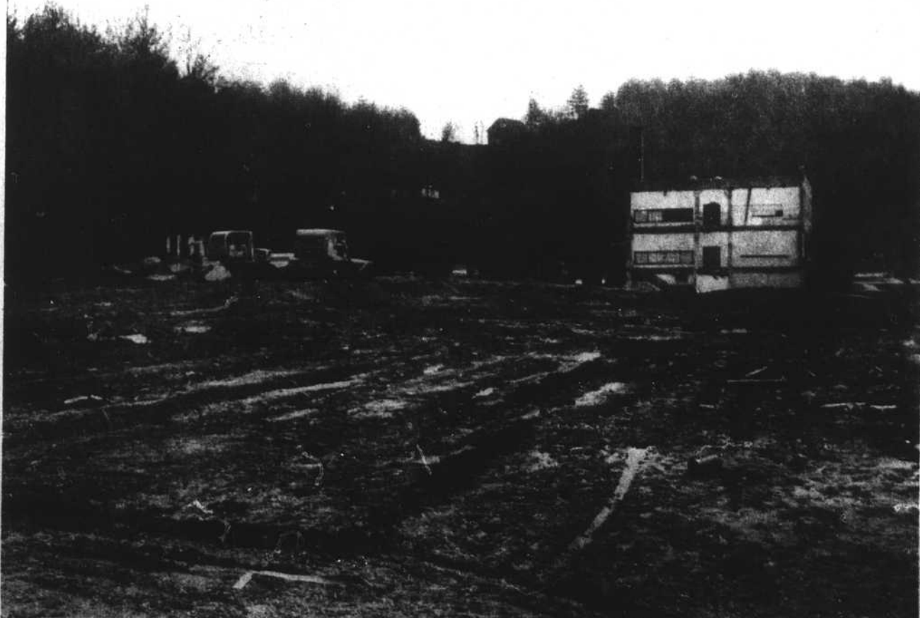
FAST WORK—This was the scene Saturday after four working days on demolition of the old Rosman High School. The building has disappeared, clearing the site for work on the new educational complex for high school students at Rosman. High School students will complete their year in the vacated elementary school facilities. (Times Staff Photo)
