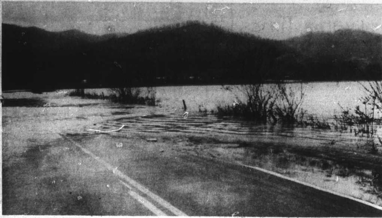
ISLAND FORD area was under water Monday morning following the heavy rains and storms of Saturday and Sunday. Hundreds of acres of bottomland was under water as the tide
