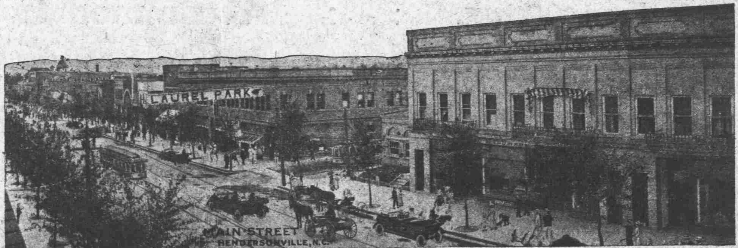
Main Business Thoroughfare, Hendersonville, N. C.
