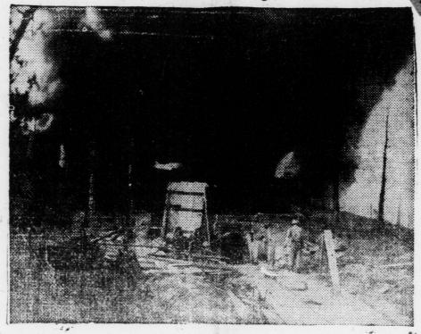
Tunneling to a depth of 30 feet below a roaring oil well near Longview, Texas, employees of the Shell Petroleum Corporation, extinguished a fire which had raged 26 days consuming approximately 10,000 barrels of oil a day. By laborious tunn eling, the fighters stopped the steady oil flow which fed the flames. It was first the attempt ever made in the Texas field to curb fire by this method.
