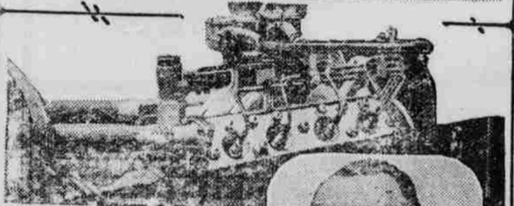
(Top)—Harold Wilson of Ingersoll and Lorna Reid of Toronto in Miss Canada IV, winner of 1935 225-inch Class races. Wilson also won 1934 races in Miss Canada III. Hulls were designed by John L. Hacker of Saginaw, Mich. (Center)—Ford racing engine showing two carburetors and Bohmaltite cylinder head used in the winner, Miss Canada IV. (Right)—David E. Anderson, Eohn engineer, who converted the Ford V-8 engine for racing purposes raising the horsepower to 140 which is exceptional
