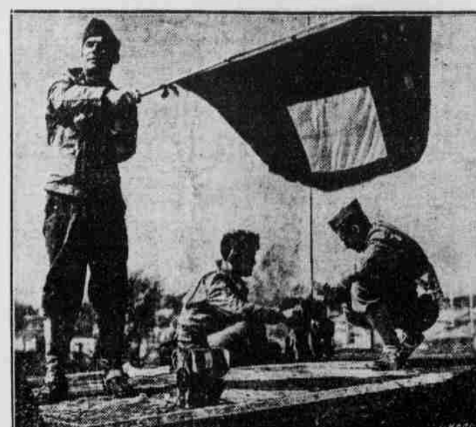
U. S. Signal Corps Photo OLDTIME WIGWAG WIGWAGS STILL—Semaphore signaling is extensively used. The wigwagger with the flag repeats the code to the walkie-talkie operators, newest members of the signalmen's crew, who are equipped with portable radio.
