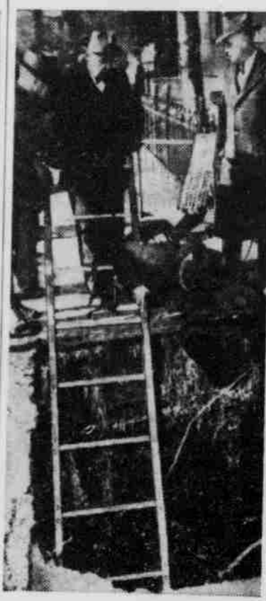
Miners dig in a 30-foot hole along a street in Pittston, Pa., for the body of Juel Ann Fulmer who was walking on the spot when the ground collapsed. She was dead when found. Workers were hampered by two subsequent cave-ins. Approximately 400 tons of debris were taken from the hole. Other cave-ins of coal mine workings have occurred previously in Pittston.
