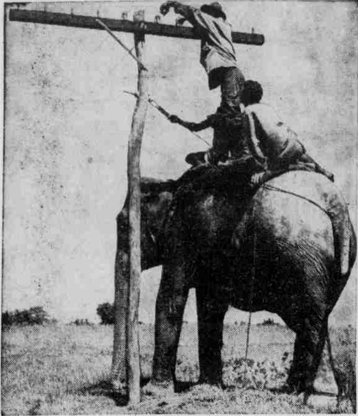
A member of the American signal construction outfit is shown repairing a line from the back of an elephant. These slow-moving, patient animals are used to very good advantage in the swamplands at Assam, India, by native and Allied troops. The signal corps, under unusual conditions, have managed to install and keep open communication lines.
