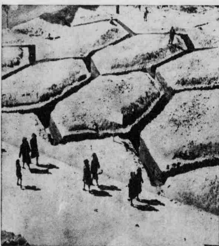
The slit trenches that cut up an area "some place in Italy" in a waffle-like pattern are being used by the Air WACs stationed near the headquarters of the 12th air force in Italy. This new type of trench is said to offer considerably more protection, and is harder to hit from air.
