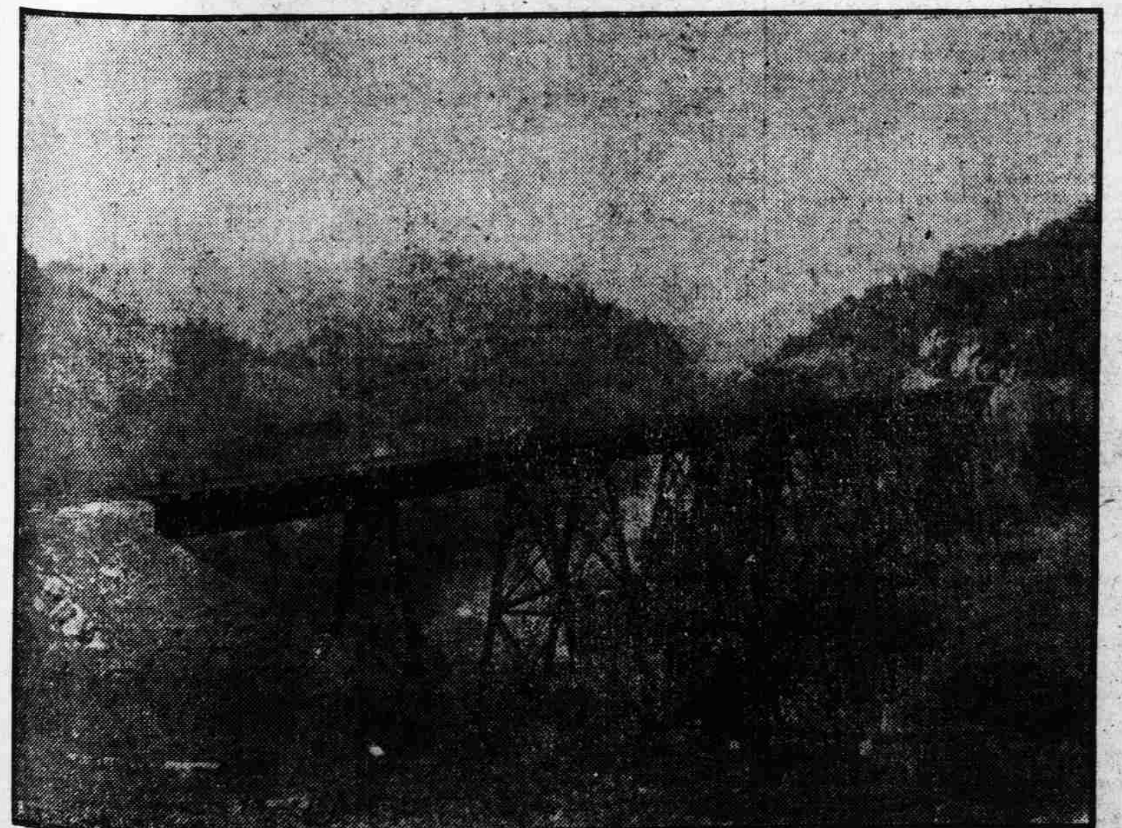
Viaduct on the C. C. & O. Railway, over Copper Creek, Scott County, Va. This viaduct is 165 feet high and 140 feet long. (On the route of The Observer's Big Excursion, July 15).
