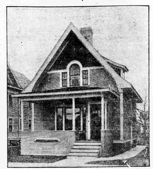
We submit for the consideration of our readers a small but neat cottage design of five rooms, the size being 20 feet wide by 24 feet deep. The cost of this house should not exters' material and labor complete, \$850; all mason work complete, \$250; painting, \$100; total cost, \$1,200. templates building the house simply with Norway pine finish on the incellar and good foundation wall.
