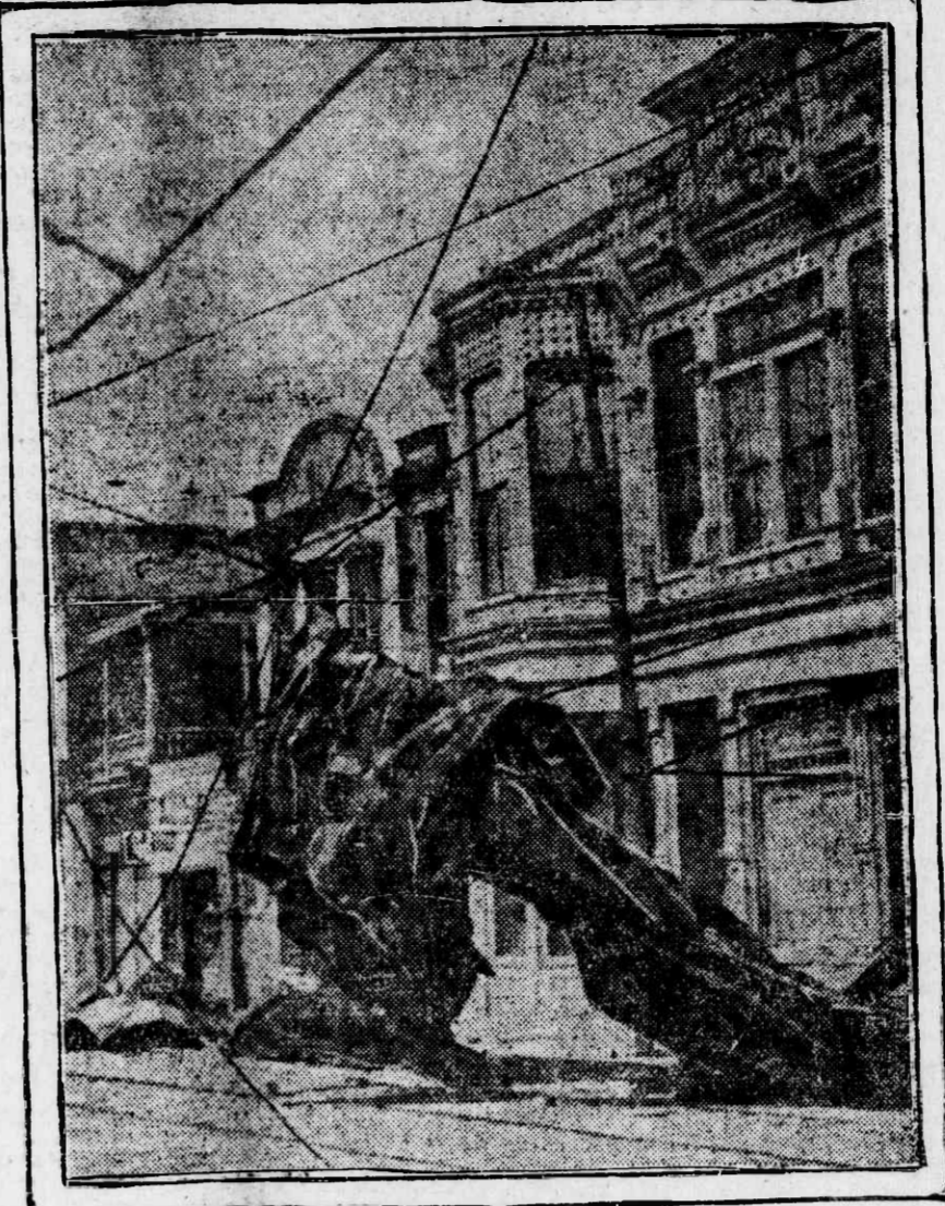
CHARLESTON AFTER STORM. Photograph showing damage done by the recent Atlantic Coast hurricane. The terrific force of the hurricane that swept up the coast may be seen in the above picture of a scene in Charleston, S. C. The trolley and telephone wires were blown down forming a network above the street, on which the roof of a house caught after it had been torn from a building. Windows were broken in by the score and the streets were littered with glass.
