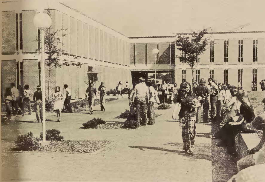
Expansion goes on. While students walk to and from their various classes, the building of the new Earth-Life Sciences Building goes on.
