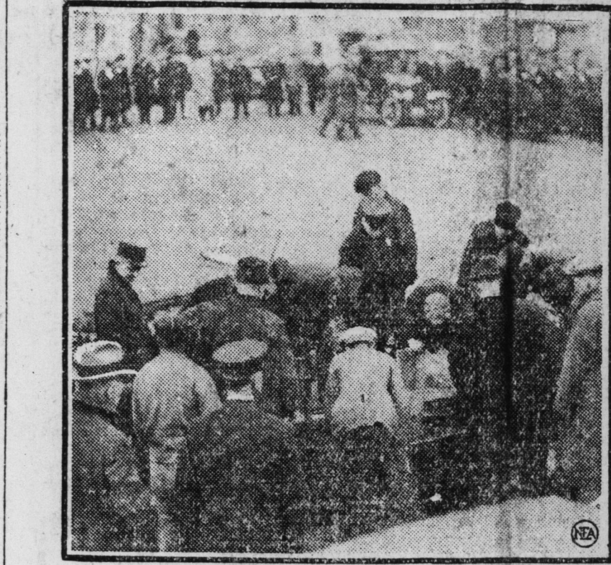
Three men were killed and two others seriously injured when they were entombed 40 feet below the street level in this sewer cave-in in Milwaukee.
