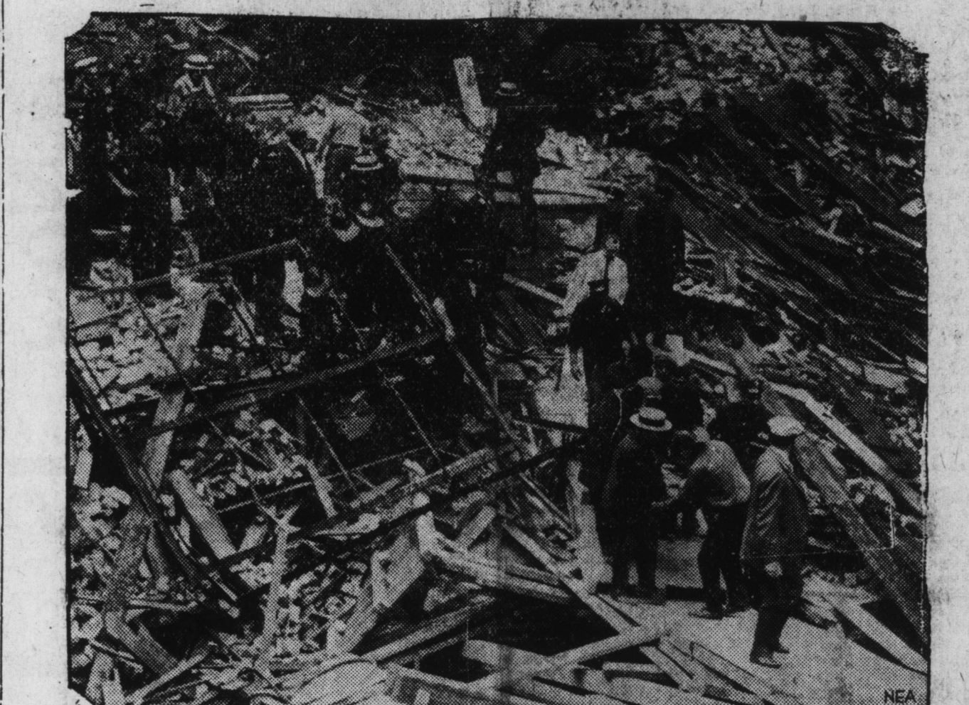
Approximately forty people were killed when the Pickwick Club, in Boston, collapsed while a dance was in progress. The picture above shows firemen and police carrying bodies from the ruins.
