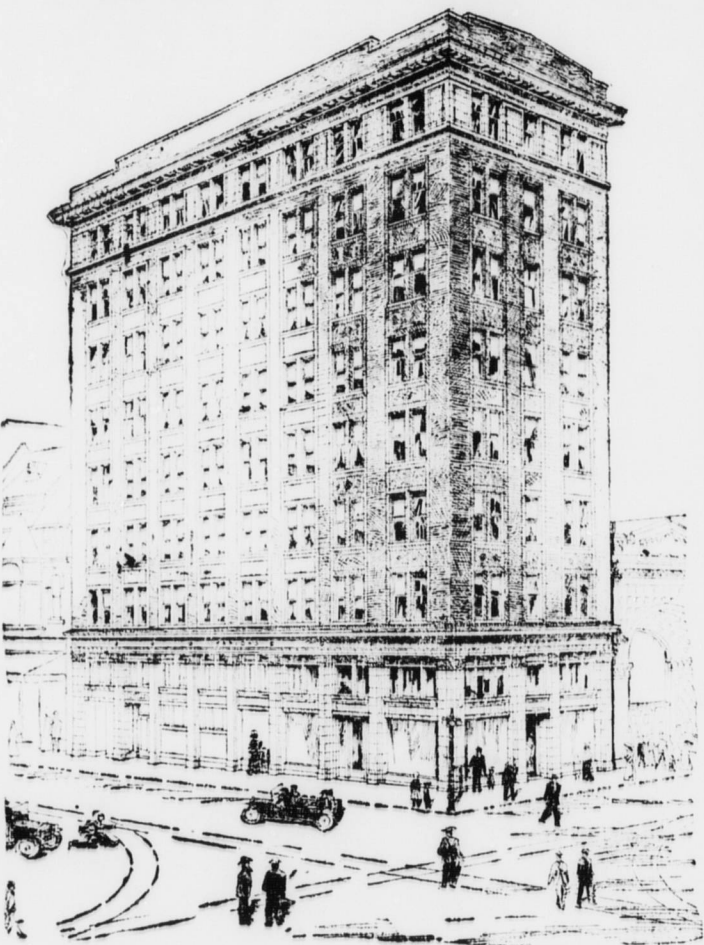
E. W. O'HANLON STORE & OFFICE BUILDING. W. H. HAYDEN - DANBURY, N. C. ESTABLISHED IN 1862.
