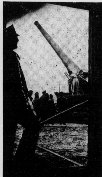
A sentry stands framed in the doorway as workmen at Baldwin Locomotive Works, Eddystone, Pa., put finishing touches on new eight-inch railway gun for U. S. army. The gun, which fires a 65-pound shell 18 miles, is the first built in a private plant since 1916.
