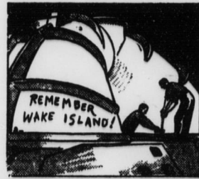
3. A sign chalked by a G-E workman on a big machine being built for war. The sign carried this challenge to fellow workers: "Remember Wake Island!"
