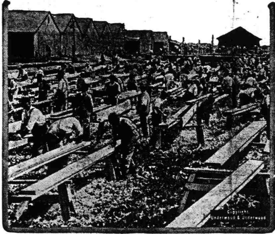
Carpenters working on new hangars at one of the aviation training schools "somewhere in the United States." Each day as more men join the air service the need for greater training camps becomes pressing. Every camp is being enlarged for the great corps of flyers Uncle Sam is training.
