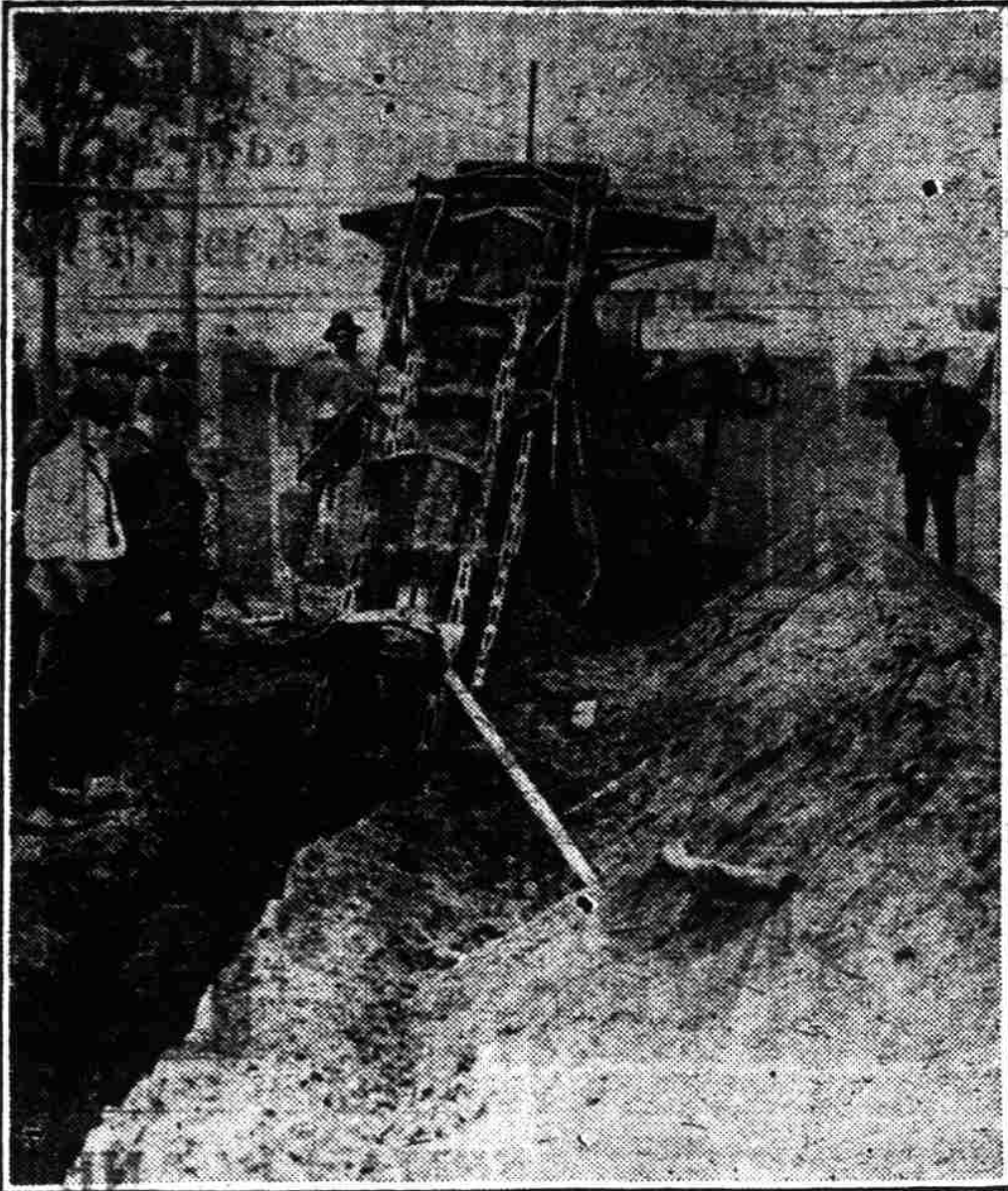
Photo by American Press Association. At the camp at Spartanburg, S. C., where the former New York guardsmen are quartered, this trench digger is used to drain the camp. Similar machines have been used in France to make real trenches.
