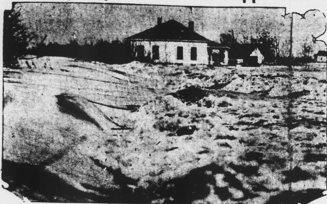
The angry, white-capped rapids shown above might well be part of the roaring torrent that rushes over Niagara Falls, but this photo was made near Jackson, Miss., where a break in the levee resulted in the waters of the Tallahatchie River inundating more than 40,000 acres of rich delta land. Despite the superhuman efforts of an army of volunteers, who labor night and day to strengthen the barriers, the tributaries of the mighty Mississippi continue to batter down all resistance, spreading watery desolation throughout the valley. Note the height to which the flood has reached on the house above.
