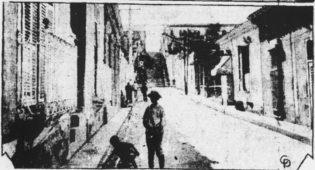
Here are two views of Santiago, Cuba, where a disastrous earthquake virtually demolished the entire city, snuffing out at least 200 lives. Almost every building in the stricken city was either razed or damaged by the quake, though it lasted but 30 seconds. Santiago, 8,000 feet above the Caribbean Sea, on the eastern tip of the island, has a population of 160,000, many of whom are Americans. Aid is being rushed by every means of transportation to the scene of the disaster. Above photos show, top, a general view of the city looking toward the harbor; lower, a typical street scene.
