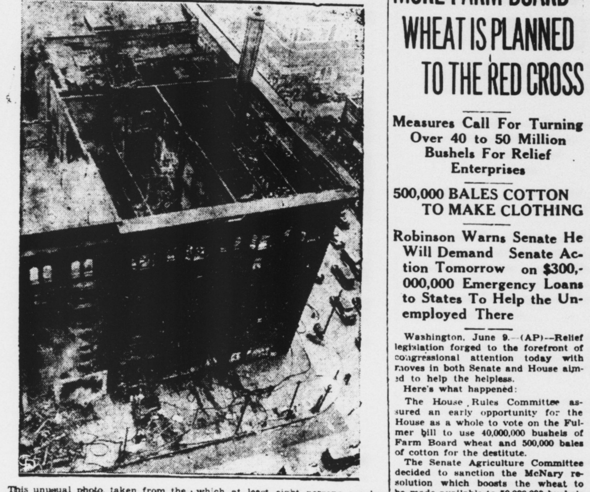
This unusual photo, taken from the roof of a nearby building, shows the charred remains of the Ellington apartments in downtown Cleveland in which at least eight persons are believed to have perished. The fire caused property damage exceeding $500,000.
