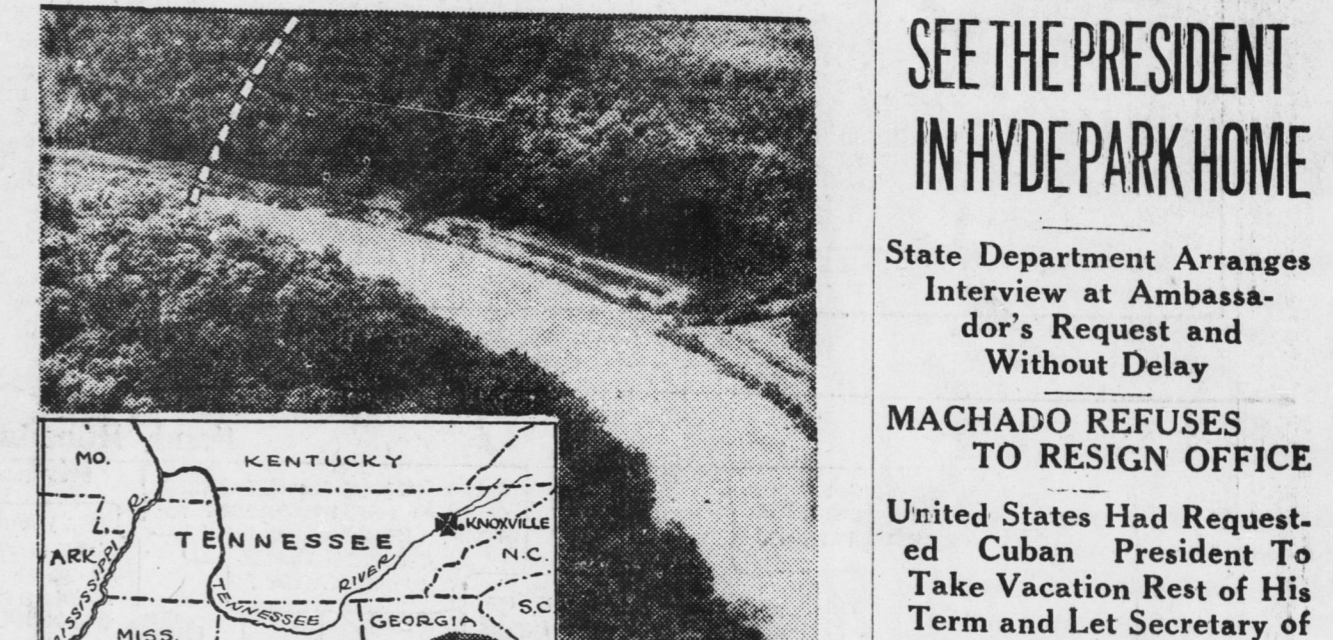
Construction of the great dam on Cove Creek, near Knoxville, Tenn., which is to be named after Sen. George Norris, leader in fight for government operation of Muscle Shoals, is being begun under the direction of (l. to r.) Dr. Harcourt A. Morgan, of Tenn., Dr. Arthur Morgan of Ohio, and David Lilienthal of Wis., shown in conference at Knoxville. Also pictured is the site chosen for the dam, which will be built at a cost of $37,000,000 as part of Tennessee Valley Authority's vast project. (Central Press)
