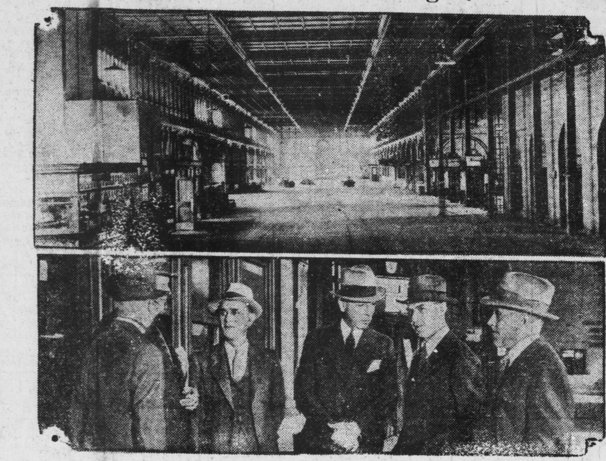
Here is a view of the upper corner of the Pennsylvania Railroad Station, Jersey City, where the Stock Exchange will be located after its move from New York, scheduled for October 3, to avoid municipal taxes.
