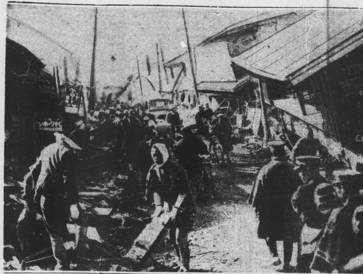
Photograph taken during a recent previous earthquake in Taihoku, Formosa, which likewise took heavy toll of lives, shows how the box-like homes of the natives are leveled to structures of cards by the tremblers. This explains the heavy loss of life. Tremblers of similar proportions caused far less damage in U. S. with its stronger buildings
