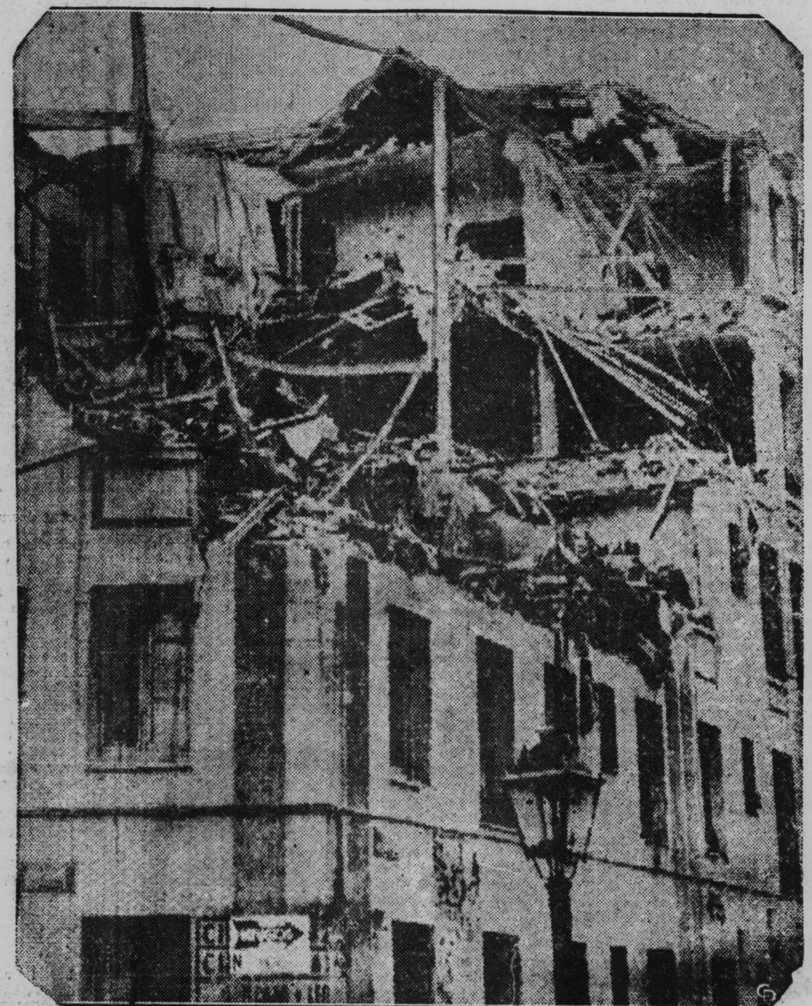
This photo, flown to London from Madrid and then radioed to America, is the first to be published in America showing the destruction wrought to the business district in Spain's capital city by rebel airplanes and shells. This particular business structure was blasted to pieces down to its second story.
