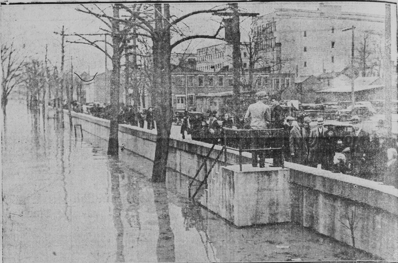
Portsmouth, O., flood wall, pictured just before continued rise of Ohio river forced water department crews to deliberately flood the business district. The flood wall is 60 feet high and was built at a cost of $1,000,000 to protect the main section of the city.
