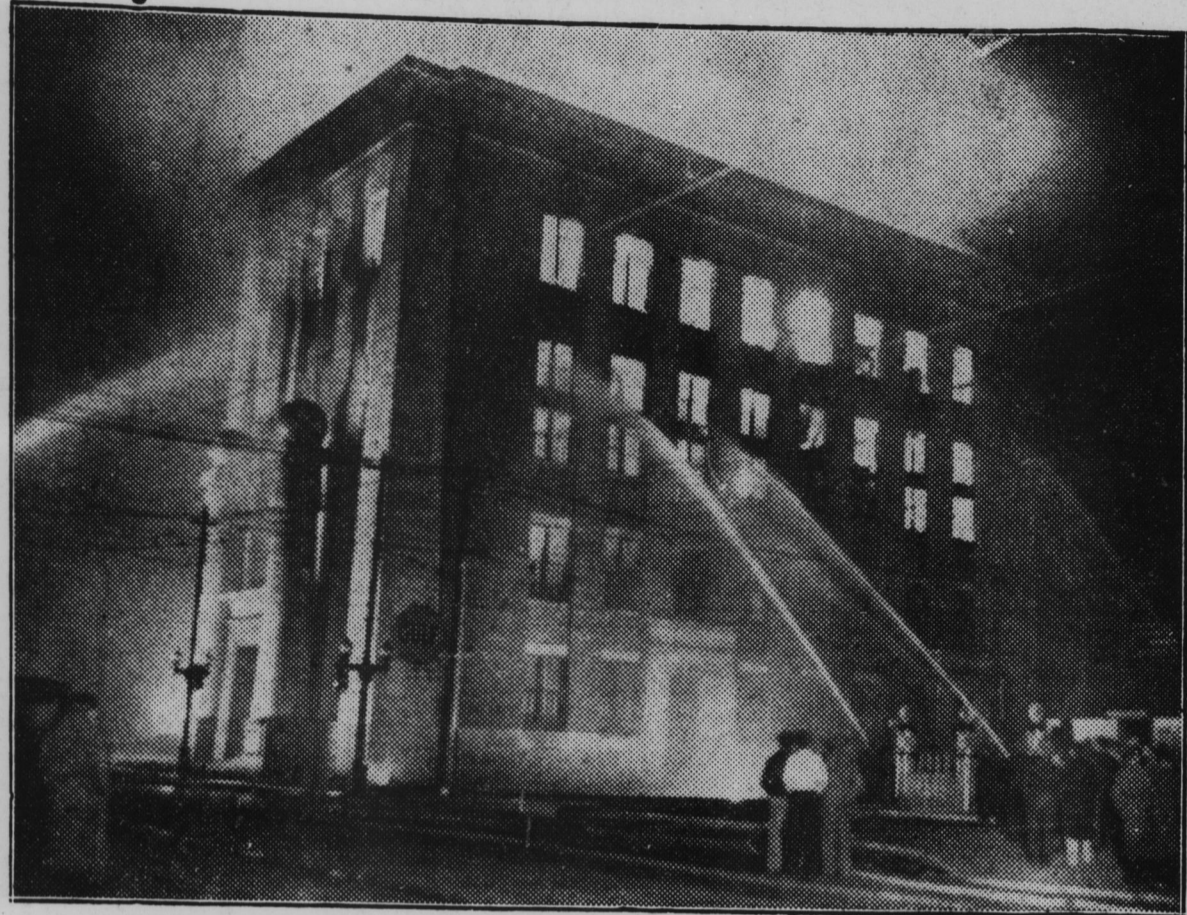
Bursting through the roof and windows almost in one spurt, a $250,000 fire is shown destroying the Masonic Temple at Charlotte, N. C. Flying embers showered on three city blocks, but principal damage aside from the Temple itself was confined to awnings. (Associated Press Photo)
